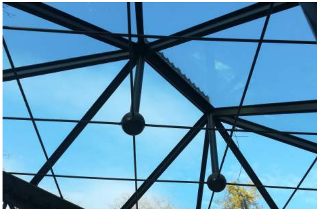
Diagonal poles connection
