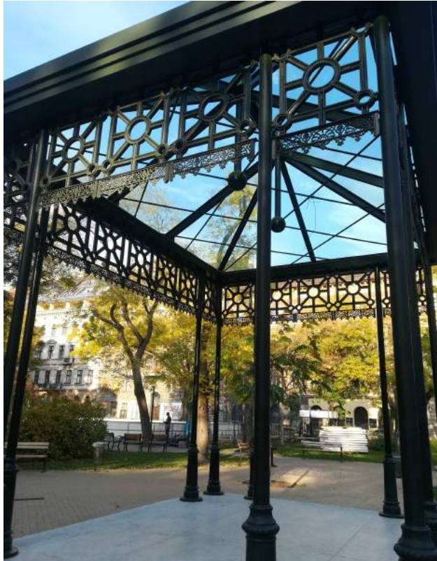
Vertical, Horizontal poles connections and three columns
